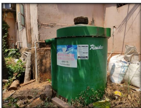
Biogas plant installed near the canteen
