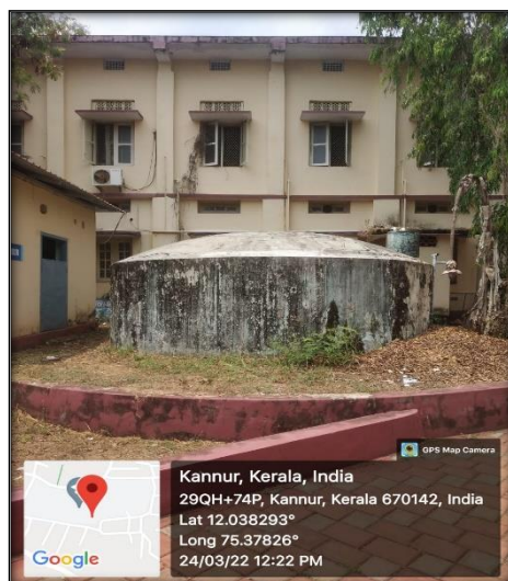
Rainwater harvesting tank of capacity 53000 L installed on the Campus
