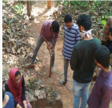
Kotoor Way Construction, Kurumathoor.
